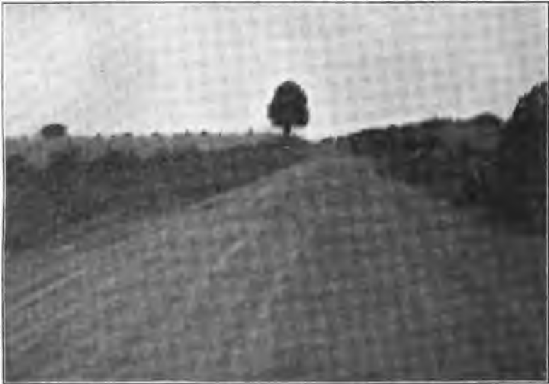
Stewartsville road, Warren Co., before improvement.
